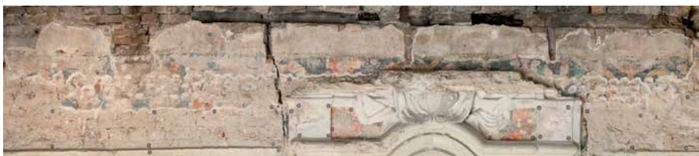
Fig. 11 Uncovered frieze in room II. State from 2013. Test windows in the chimney piece. Phot. W. Holnicki
